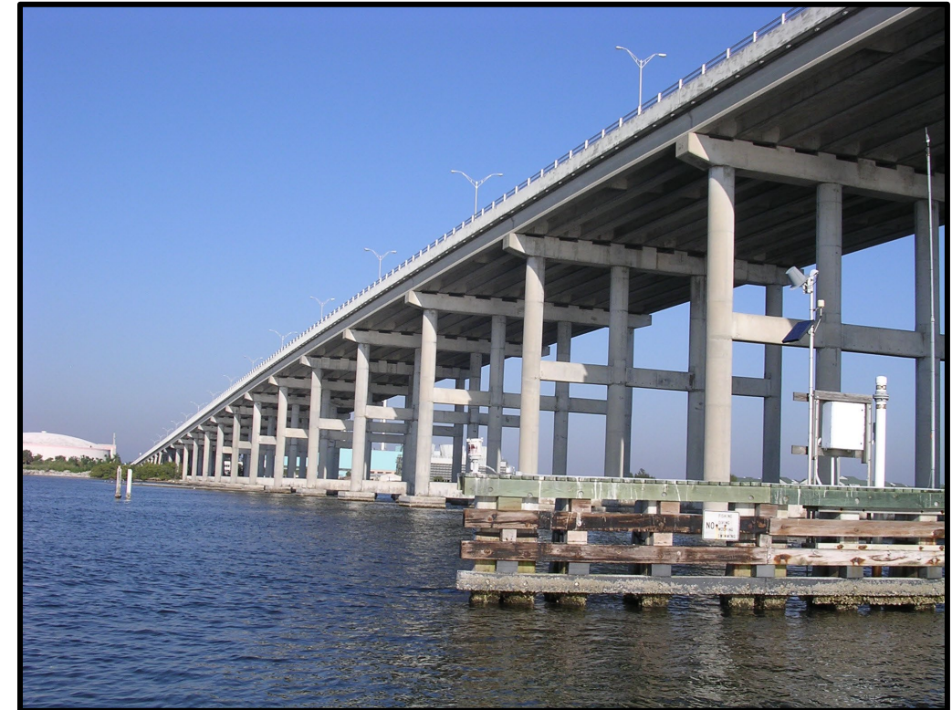
SR-656/17 th Street bridge looking west. (pre-construction)
